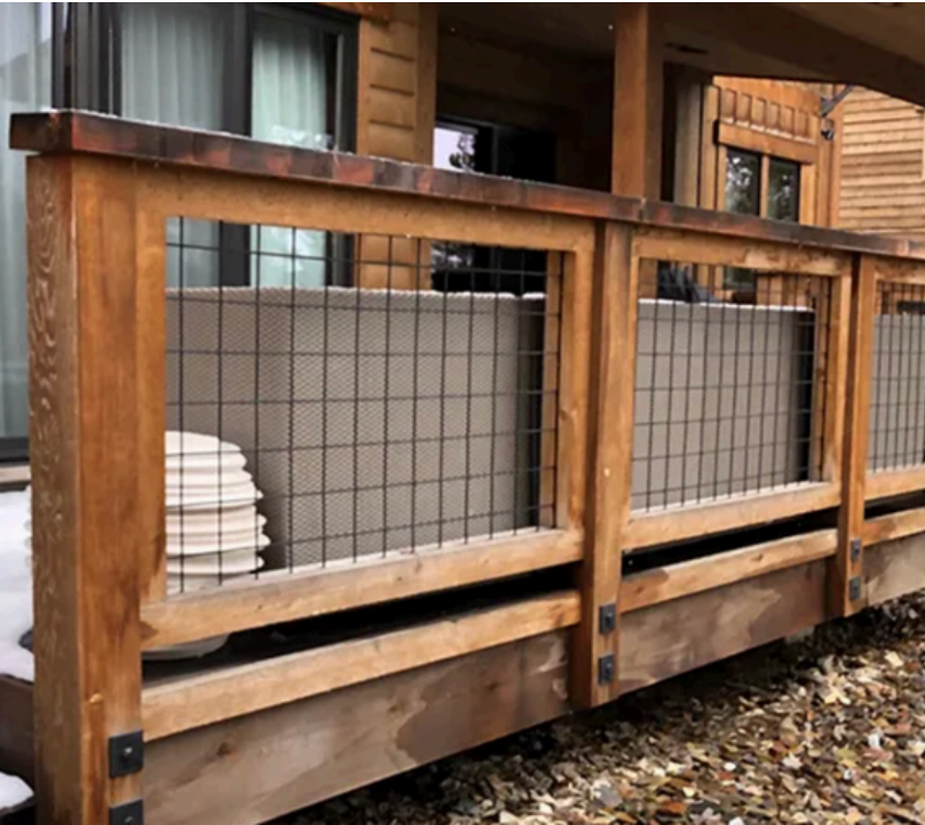
Railing: Douglas fir posts stained SW 3532 Hill country exterior semi transparent stain with hog wire
